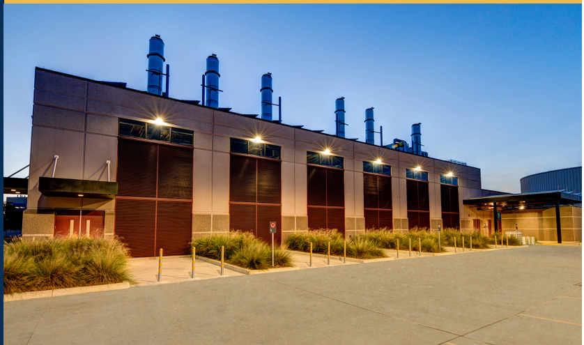
Combined Heat & Power Plant Michael E. DeBakey VA Medical Center, Houston, TX
