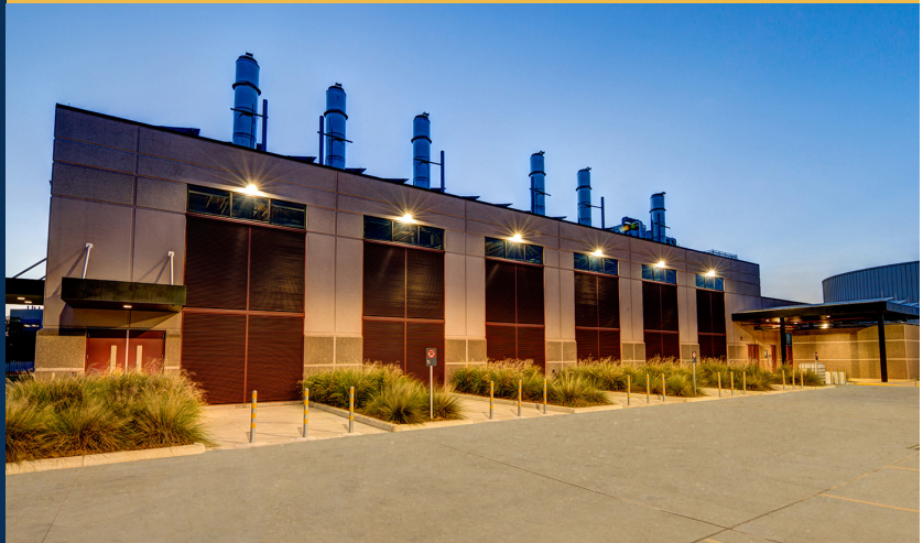
Combined Heat & Power Plant Michael E. DeBakey VA Medical Center, Houston, TX
