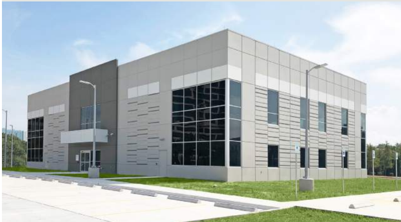
New Administration Building Michael E. DeBakey VAMC, Houston, TX
